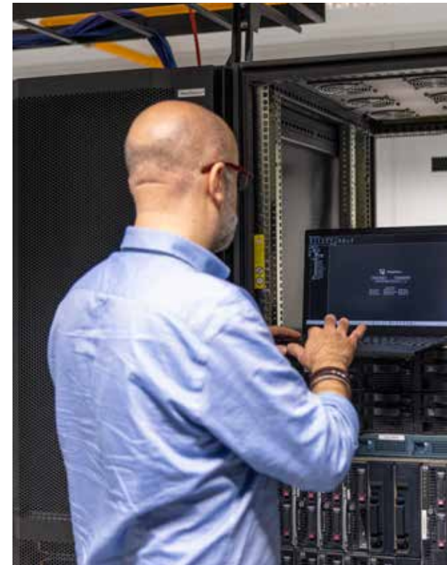
Smart Buildings e Data Centers
