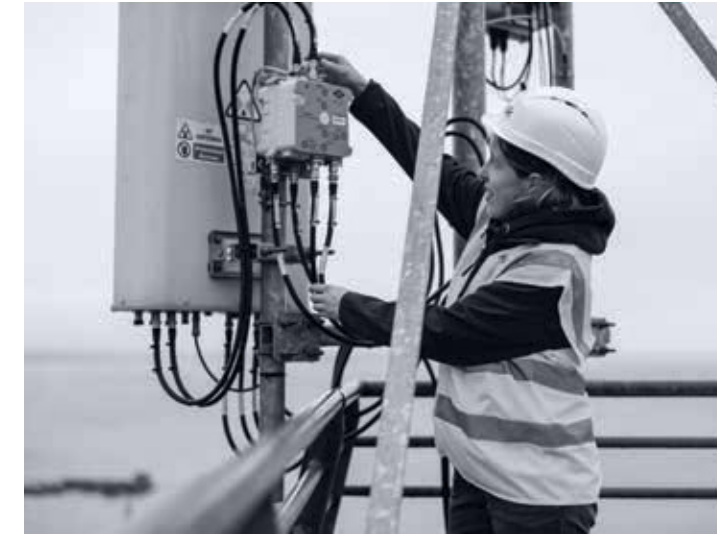
Installation of equipment
